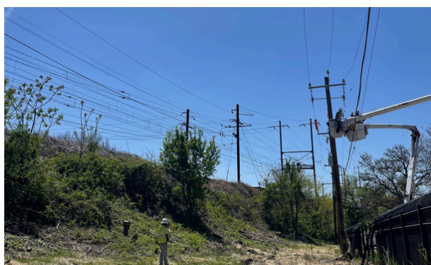
Delmarva undergrounding utilities prior to the BGE Tower Relocation Project.
