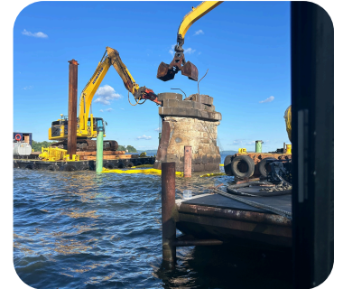
Pier 6 being removed from the river
