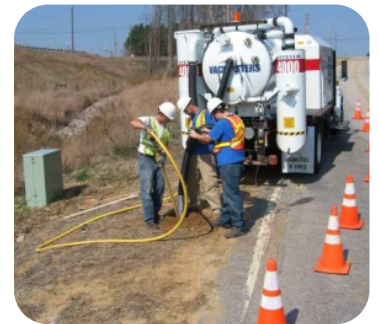
Identification of subsurface utilities
