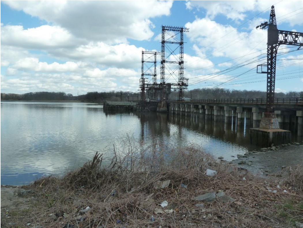
Photograph 3. View of Amtrak Pelham Bay Bridge looking northeast (4/20/22)
