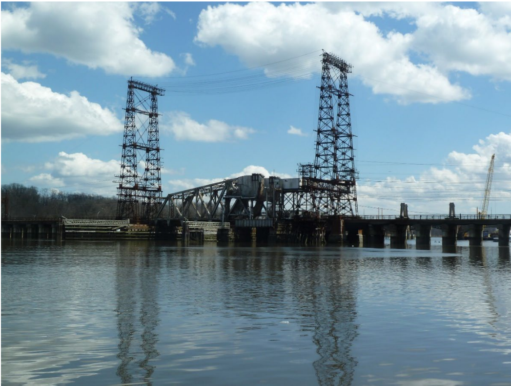
Photograph 2. View of Amtrak Pelham Bay Bridge looking east (4/20/22)
