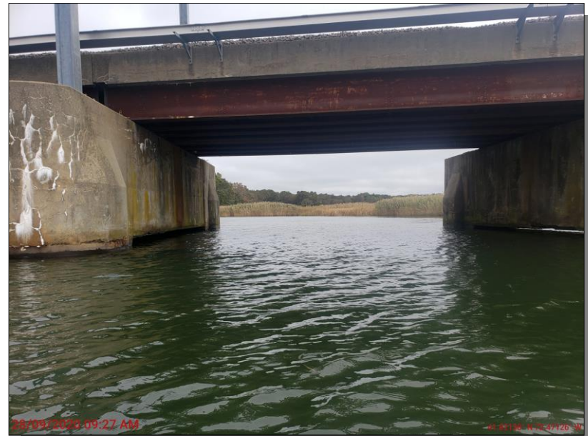
Photo 20: Amtrak bridge over the Lieutenant River; facing northeasterly
