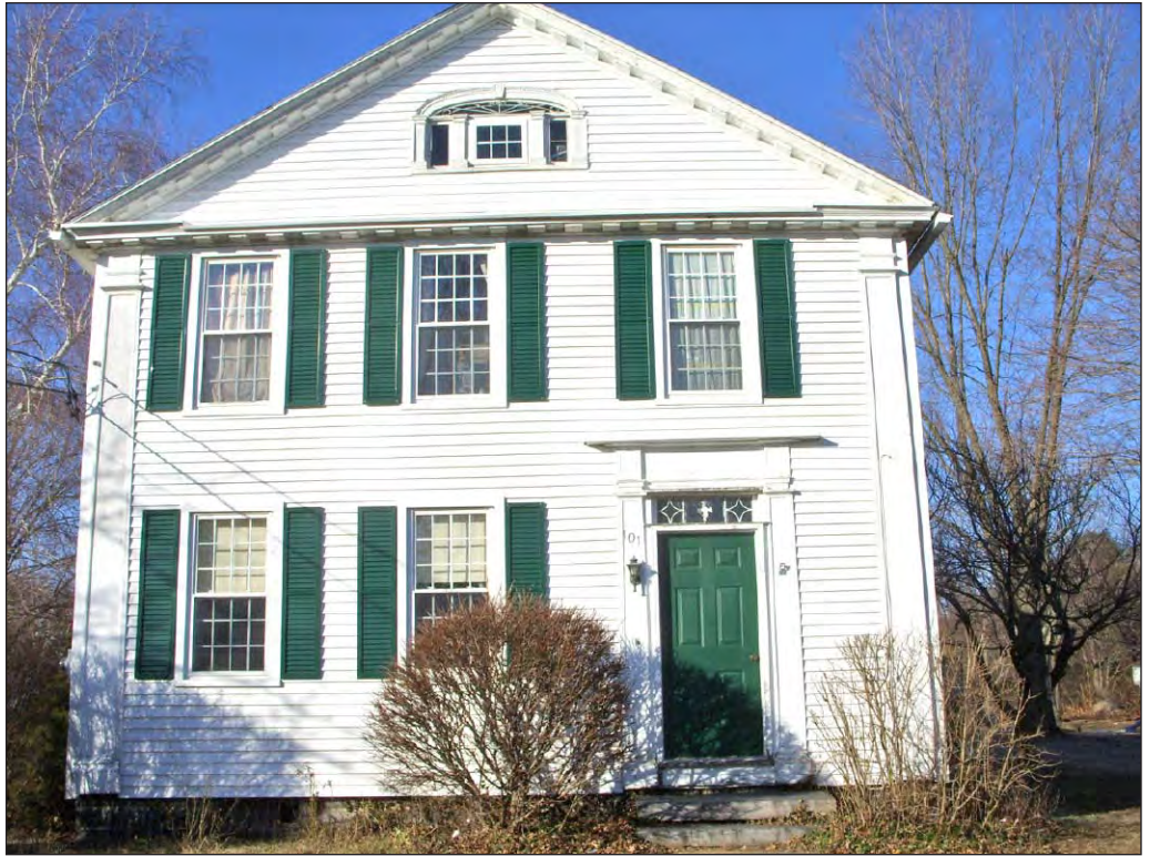
The Federal-style house at 101 Ferry Road in Old Saybrook, roughly 700 feet north of the project site, is a front-gable structure with a denticulated raking cornice and a Palladian window in the gable tympanum. It is clad in wood clapboard, has windows containing twelve-over-twelve-light double-hung sash, and retains its original pilasters and door surround.
