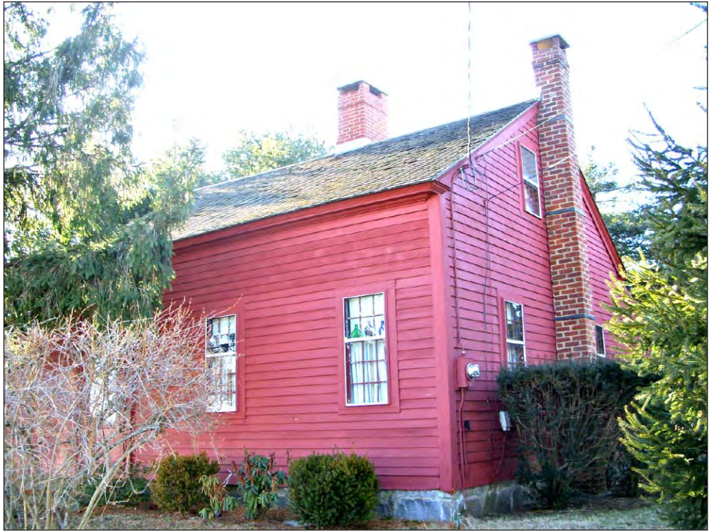
A view of the front (east) and north facades of the single-story Cape Cod-style house at 9 Clark Street in Old Saybrook; located roughly 400 feet north of the project site. The small ca. 1800 clapboard-clad "half house" has a stone foundation, a central brick chimney, and six-panel wood door. Its roof is clad in wood shingles and the windows contain six-over-six-light double-hung sash.
