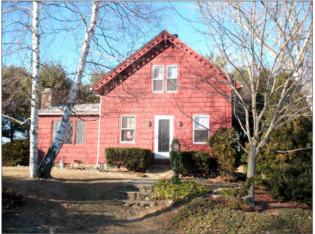
On the north side of Ferry Road in Old Saybrook (just less than a quarter mile northwest of the project site) the house at 61 Ferry Road displays elements of the Gothic Revival style. The front-gable wood-frame structure is clad in wood shingles. Its gable is ornamented with decorative quatrefoil vergeboard and a drop finial. 6
