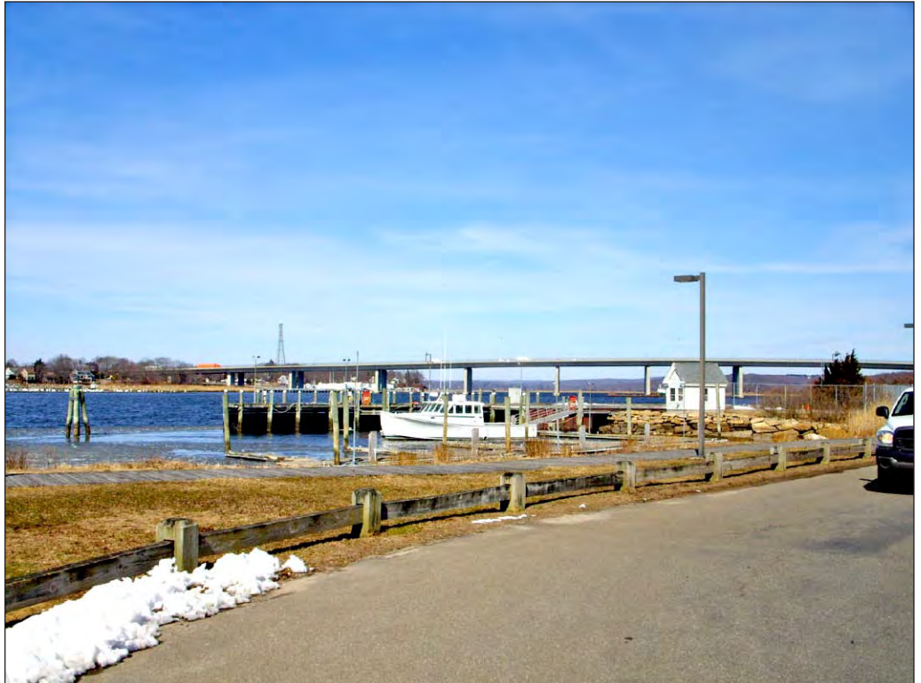
Looking northwest from the Ferry Landing Park in Old Lyme, a view of the Connecticut River, and the Baldwin Bridge. 13
