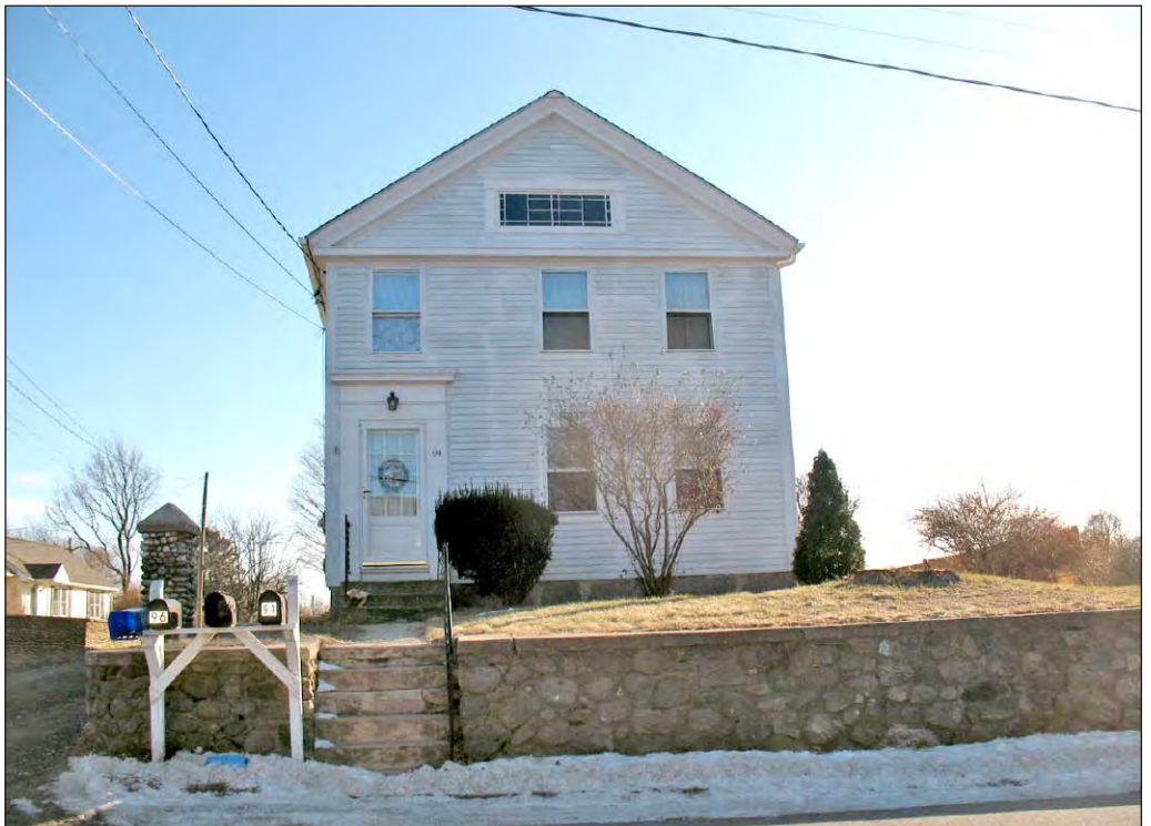
The house at 94 Ferry Road in Old Saybrook, roughly 500 feet north of the project site, is a late Federal-style house with a raking cornice, classical door frame, and a decorative gable window. It is clad in wood clapboard. Most of the windows have been replaced with modern sash. 7
