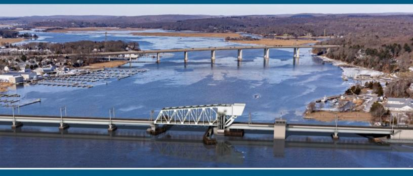
Amtrak® is building a new, modern, two-track, electrified, movable bridge to replace the existing Connecticut River Bridge. Join us to learn more about the planned construction activities and how Amtrak is improving future service reliability for passenger rail customers and local community maritime operations.
