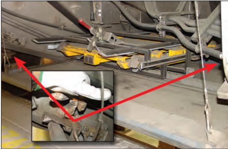
Figure 1-12 – Lower storage compartment latches and safety cables
