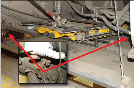
Figure 1-12 – Lower storage compartment latches and safety cables
