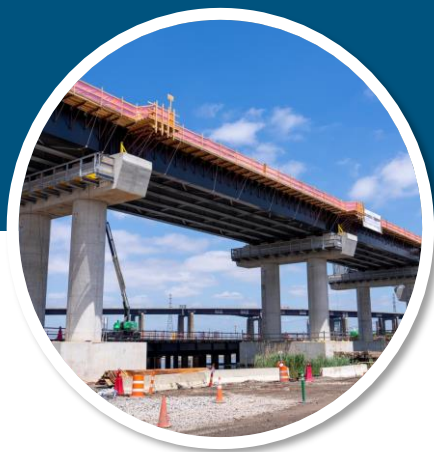
Portal North Bridge 75% complete
