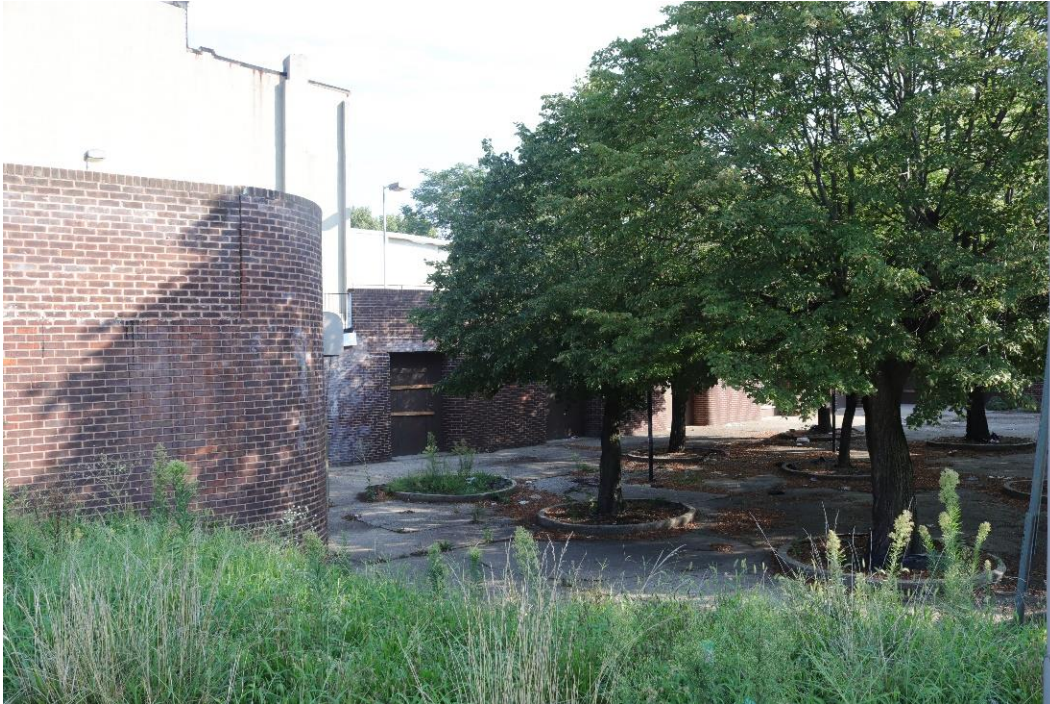
Photo 5: Southeast Elevation Facing the Courtyard, Looking Northwest
