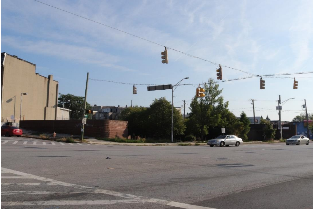
Photo 1: 920 W. North Avenue, Southwest Elevation and Southeast Façade, Looking Northeast
