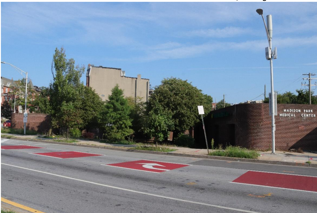
Photo 4: Southeast Elevation and Courtyard from W. North Avenue, Looking North
