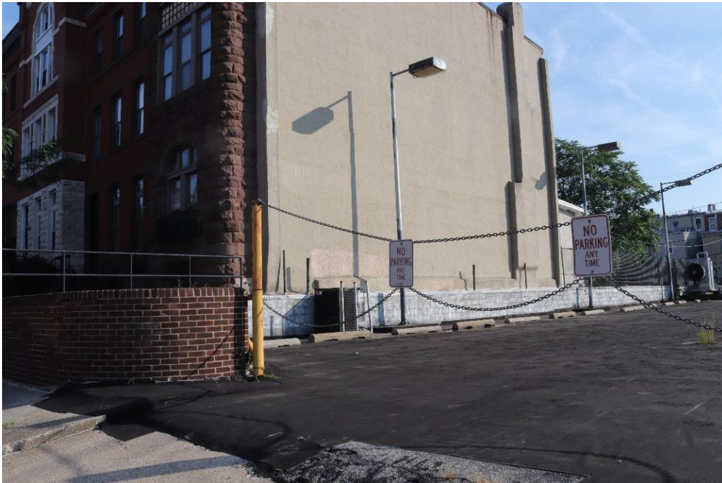
Photo 12: Northwest Elevation from Driveway, Looking Northeast
