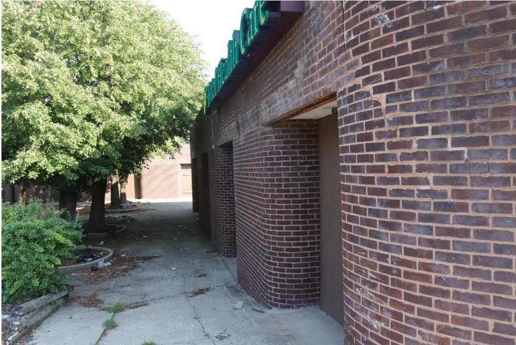
Photo 9: Southeast and Southwest Elevations Facing the Courtyard, Looking Northwest
