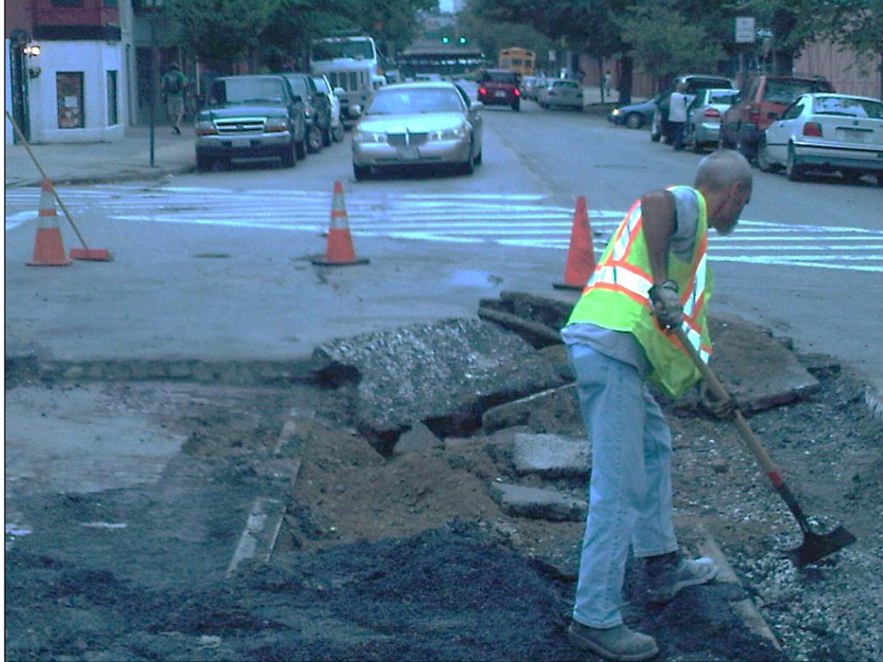
Figure 6: Intact Streetcar/Trolley Tracks, as exposed in street.
