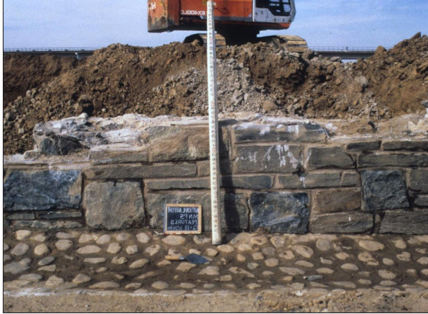
Figure 8: Intact Masonry Foundation and Cobble Paving, as exposed in excavation.
