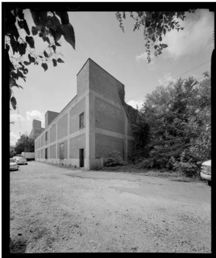
Photo 3: 2150 Harlem Avenue warehouse to be demolished as originally intended. View looking southwest. Credit: Renee Bieretz, photographer, September 2021
