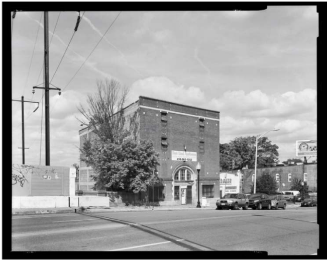
Photo 1: 2126 Edmondson Avenue, commercial building to be acquired and maintained. View looking northeast. Credit: Renee Bieretz, photographer, September 2021
