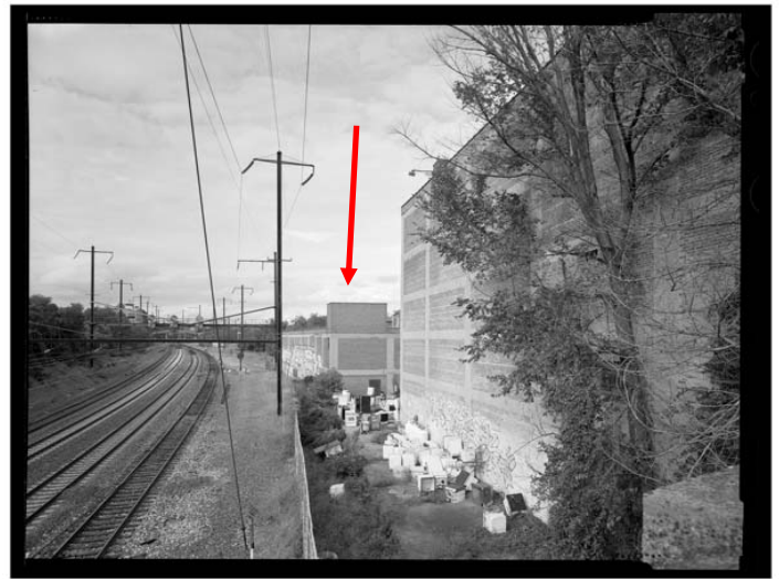
Photo 4: 2150 Harlem Avenue, warehouse. View looking north/northeast. 2126 Edmondson Avenue commercial building in foreground. Credit: Renee Bieretz, photographer, September 2021
