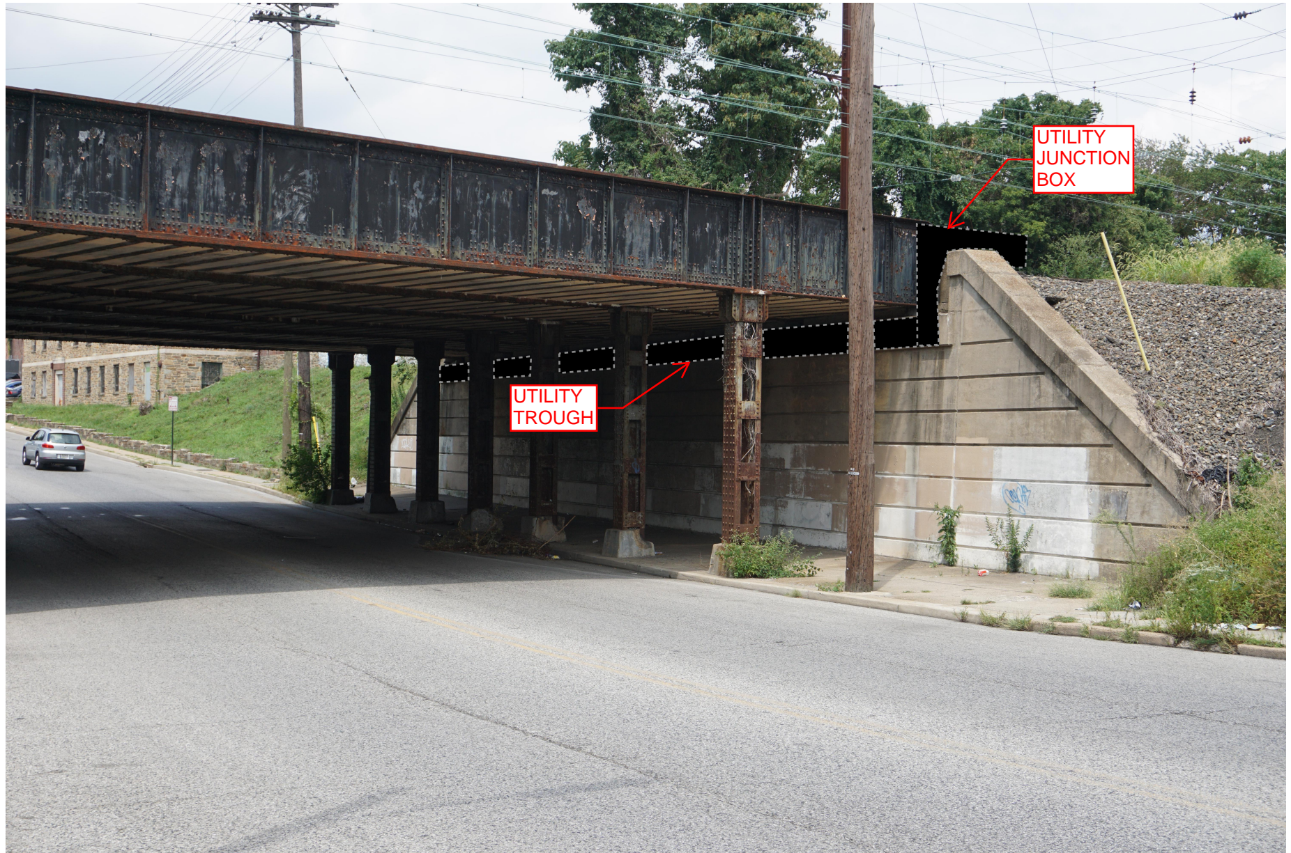
Rendering of the Utility Trough and Junction Box Mounted on the North Abutment of the North Franklinton Road Bridge Carrying the B&P / Philadelphia, Baltimore and Washington Railroad over North Franklinton Road (UG 98.95), view looking north.
