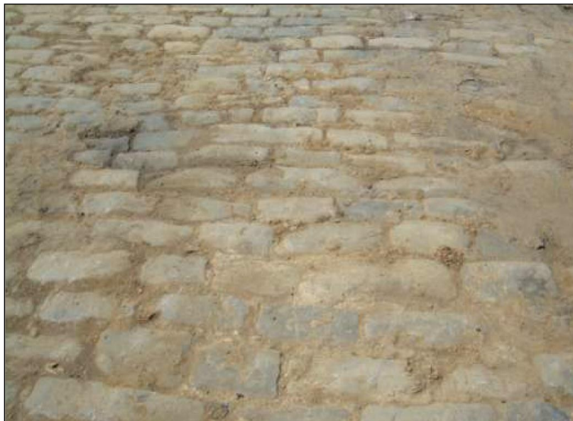
Figure 7: Intact Stone Block Paving, as exposed in excavation.
