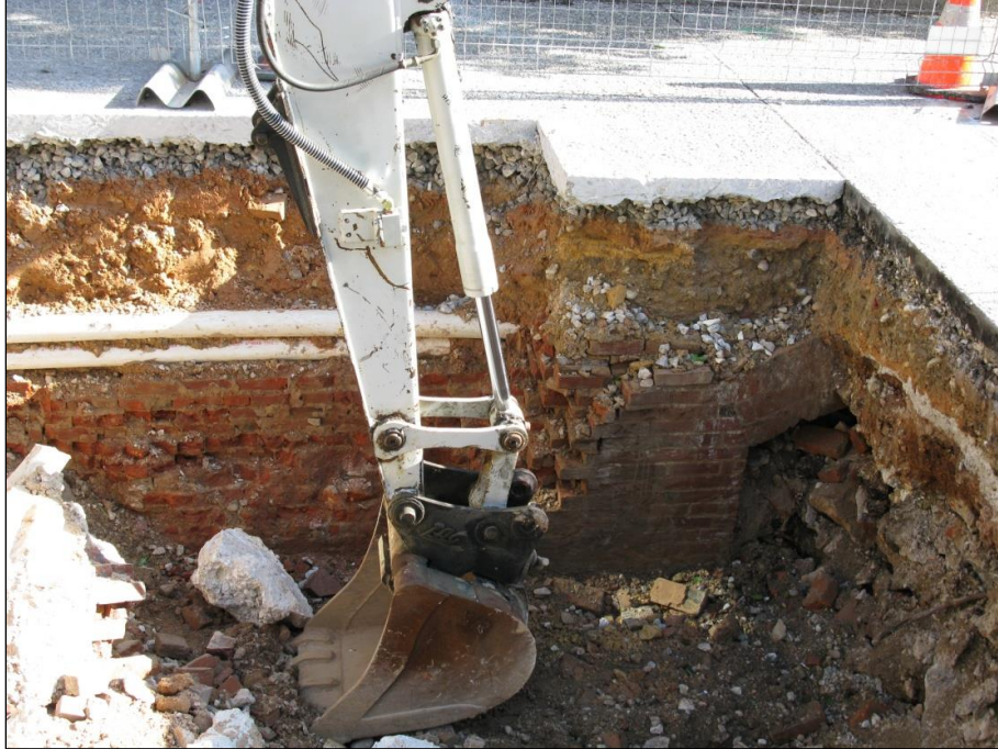
Figure 9: Intact Brick Foundation, as exposed in excavation.
