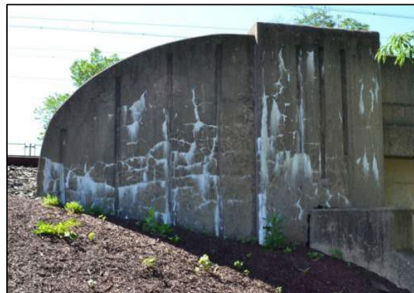
Plate 7: Cheek wall (typical), West Mulberry Street bridge.
