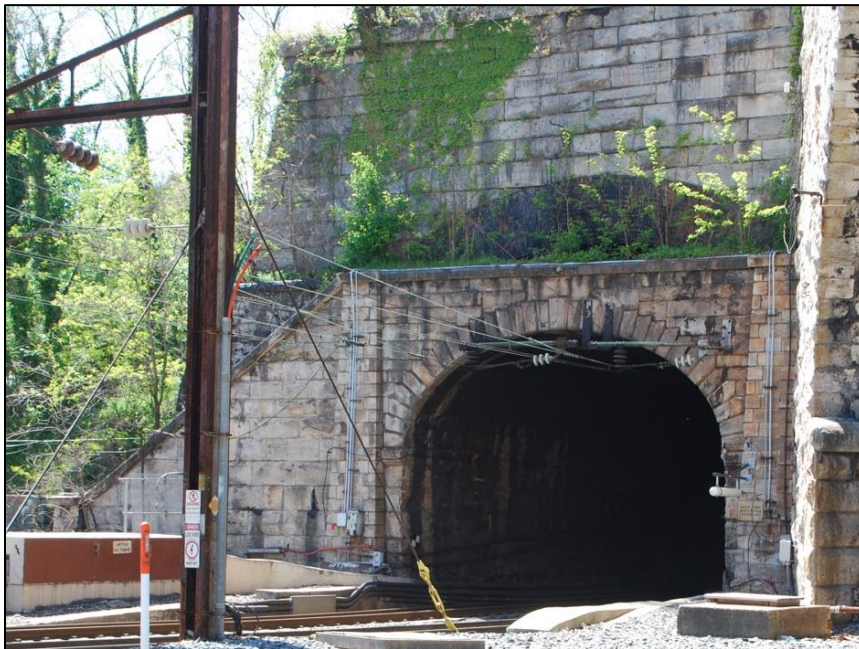
Plate 33: Existing north portal.
