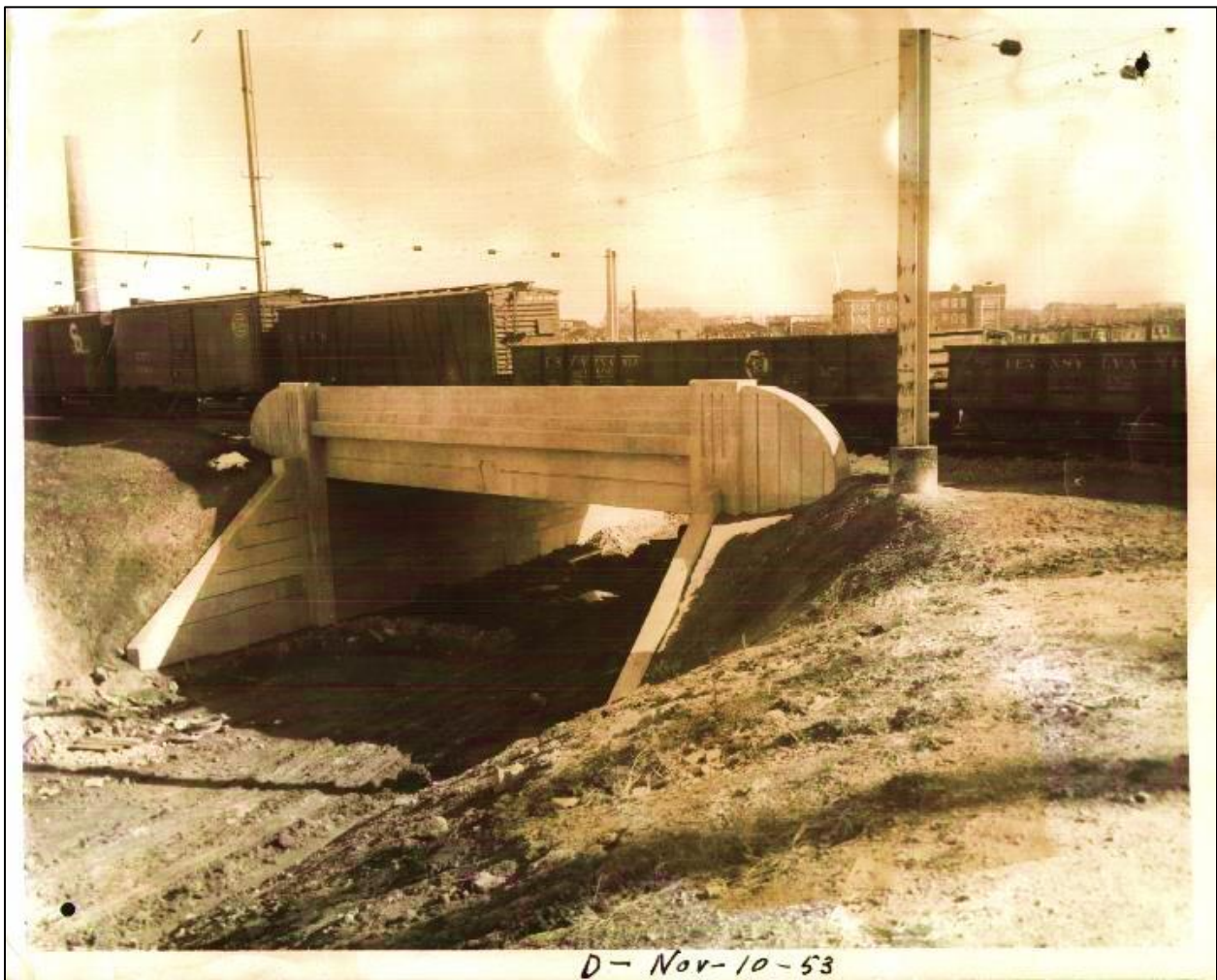
Plate 21: Historic photograph of the 1953 construction of the bridge over West Mulberry Street.
