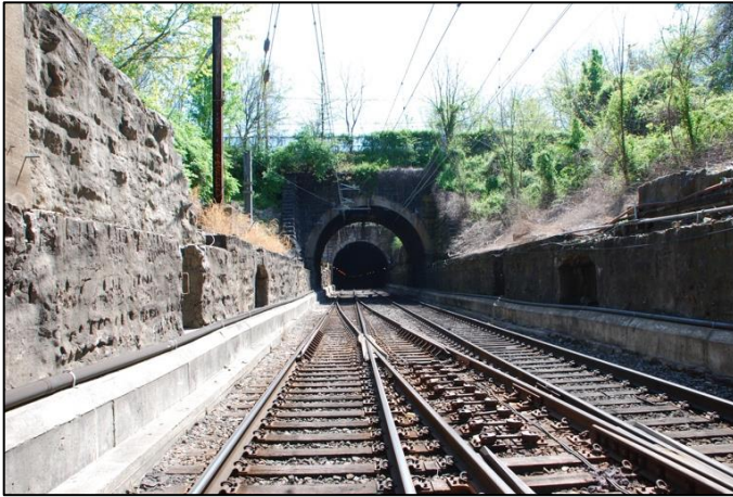
Plate 28: Typical coursed ashlar stone construction along the existing B&P alignment.
