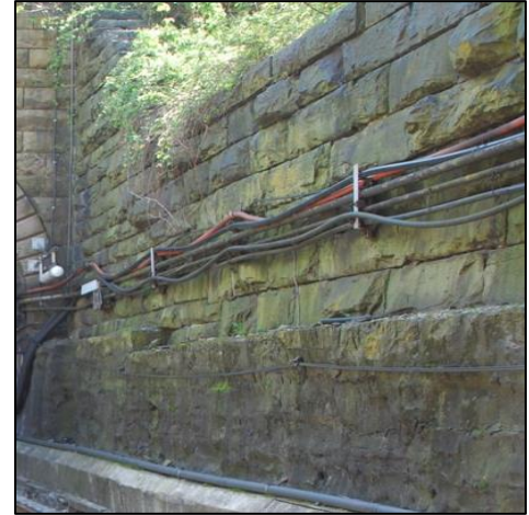
Plate 28: Typical coursed ashlar stone construction along the existing B&P alignment.
