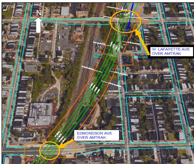
Figure 3: Two bridges carrying local roads (Edmondson Avenue and West Lafayette Avenue) over the rail line.
