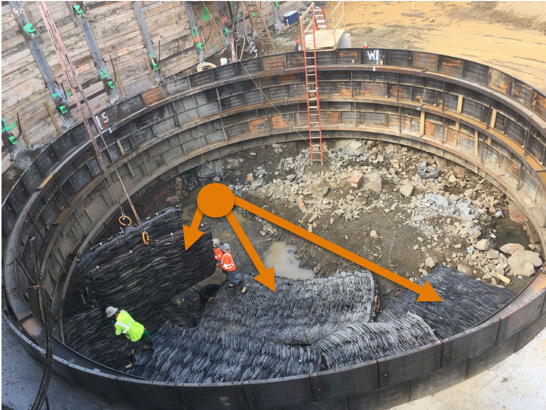
Blast Mats placed prior to round initiation
