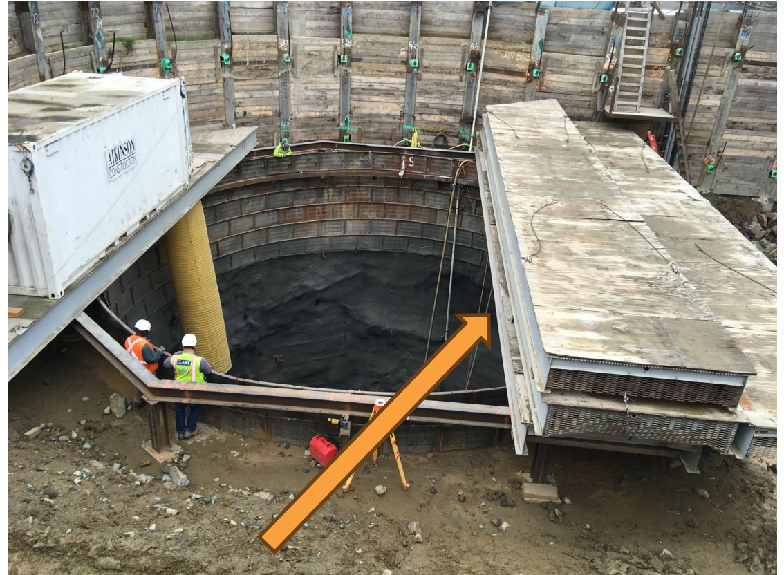
Shaft covers placed prior to round initiation
