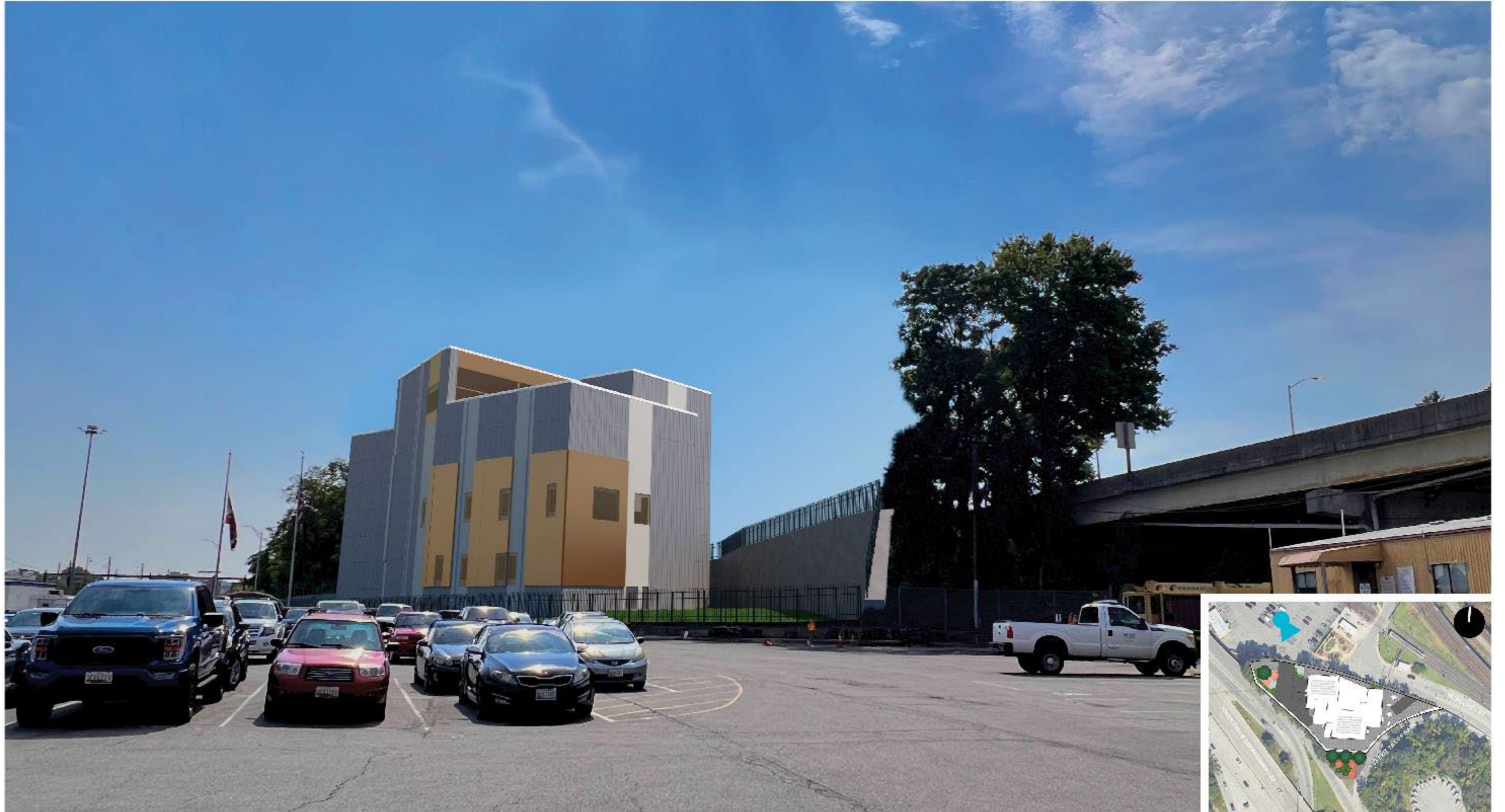
View at MTA Facility Parking Lot
