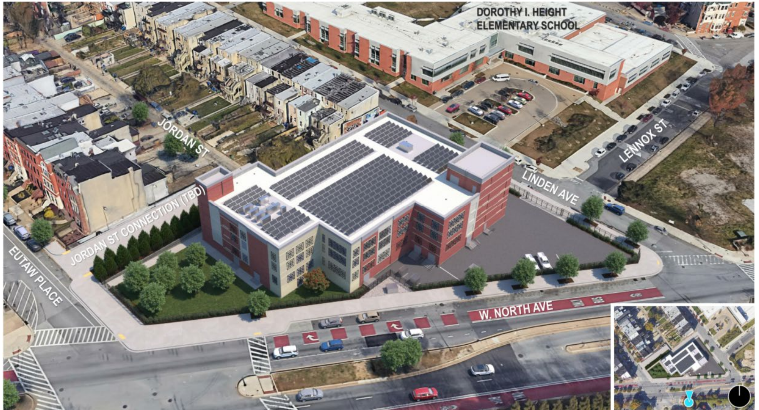
Aerial View at W. North Avenue
