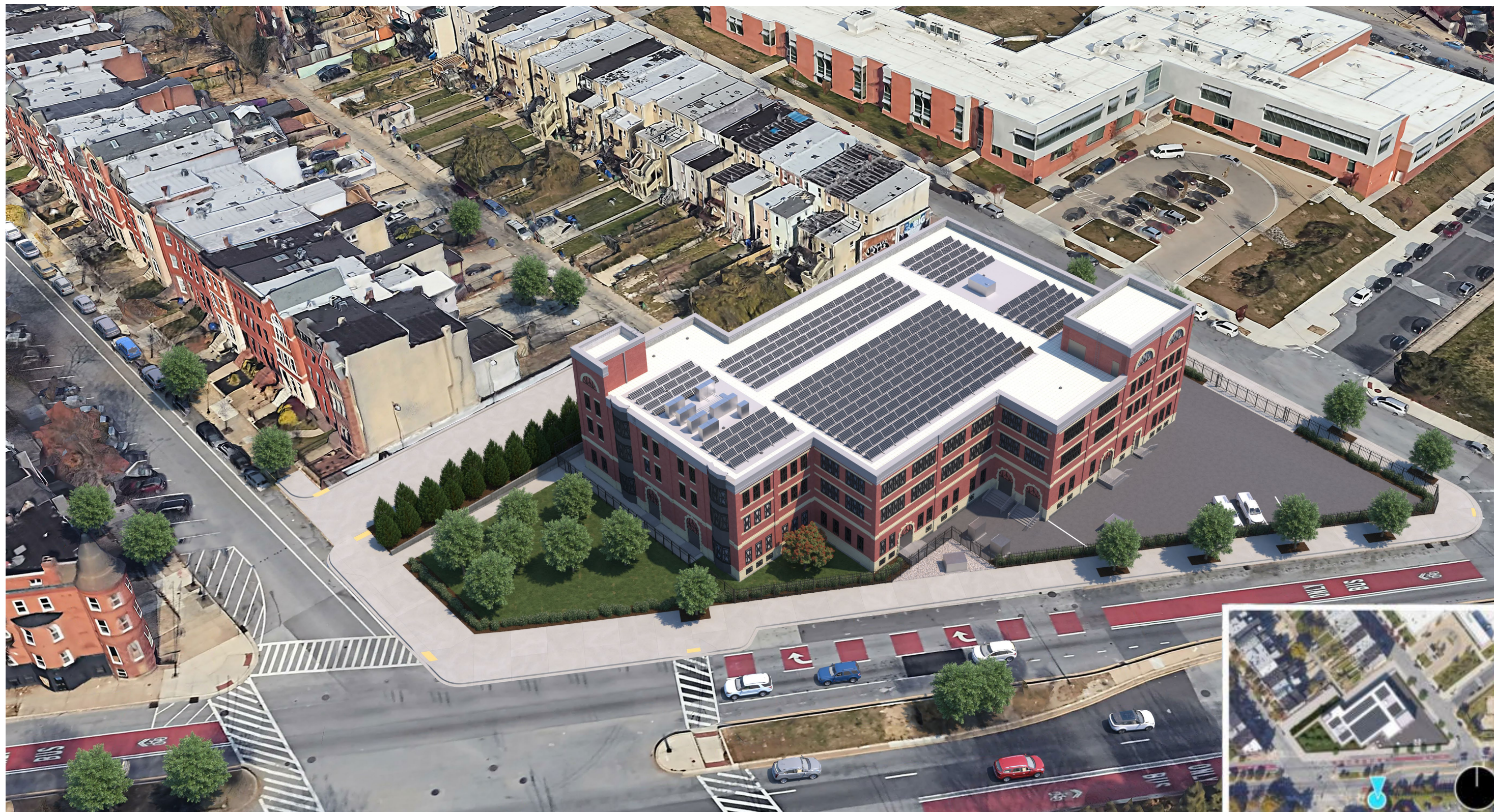
Aerial View at W. North Avenue
