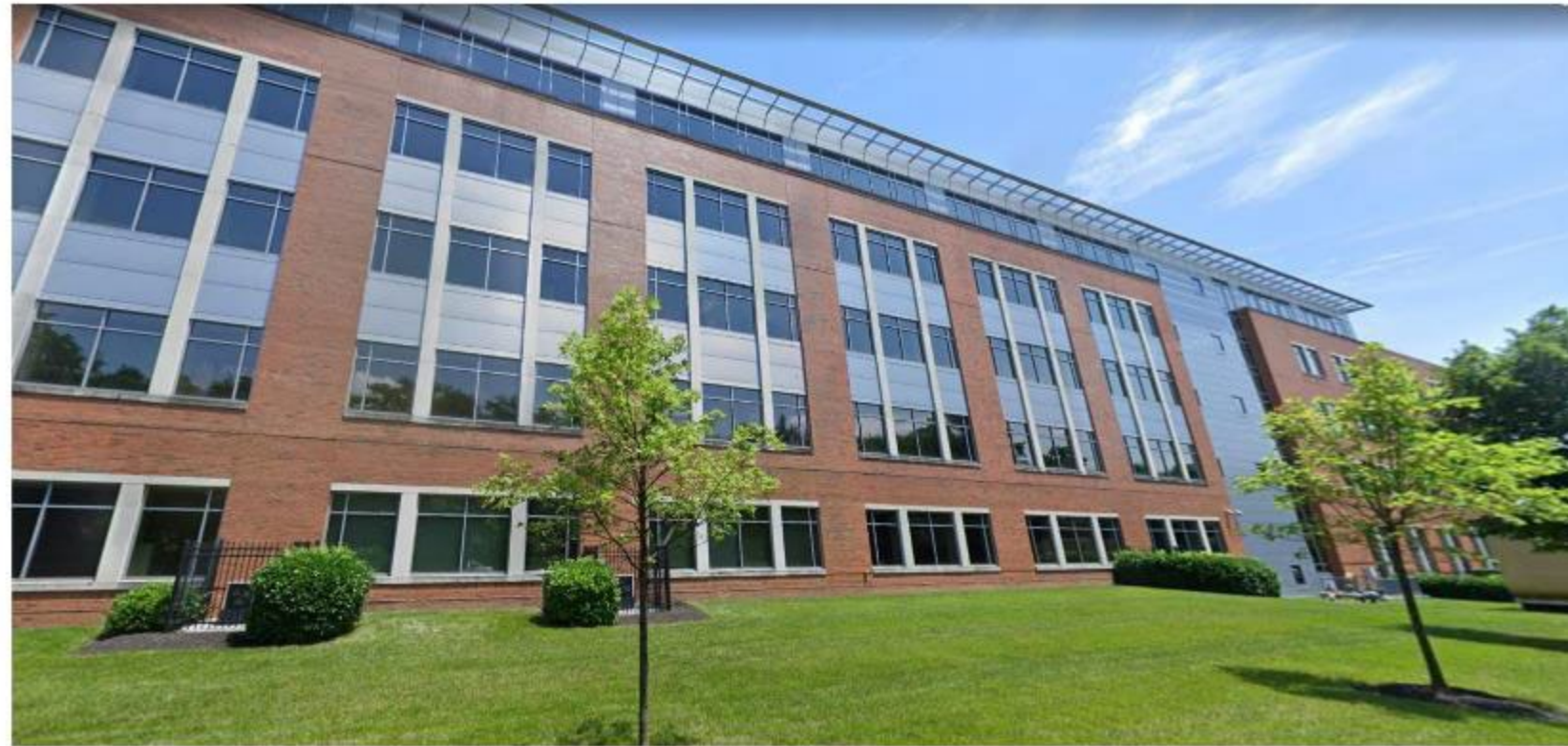
HEALTH & HUMAN SERVICES BUILDING (LOOKING EAST; BETWEEN W. NORTH AVENUE & WHITMORE AVENUE)
