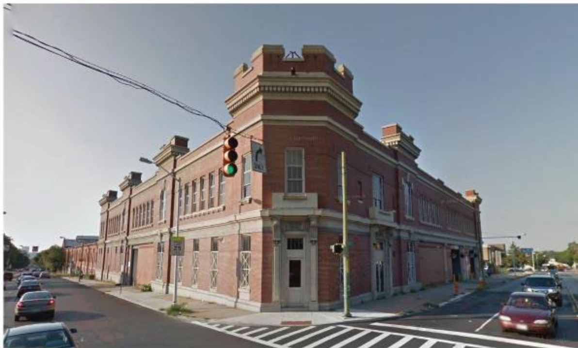
PARK TERMINAL FACILITY (LOOKING SOUTH; BETWEEN N. FULTON AVENUE & DRUID HILL AVENUE)
