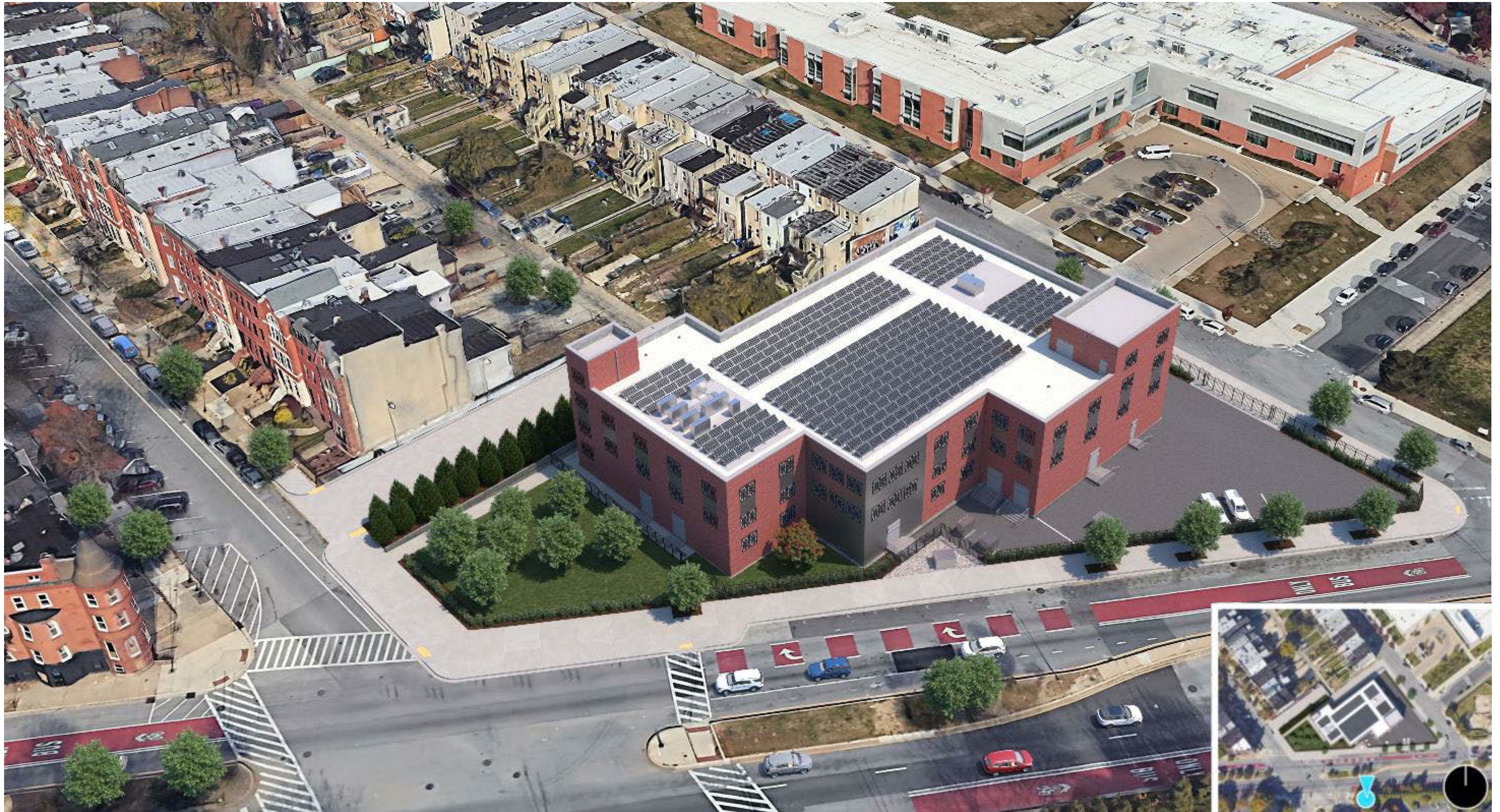
Aerial View at W. North Avenue
