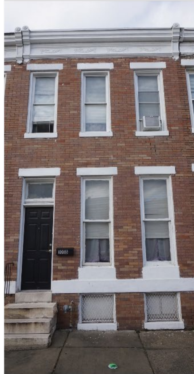
N PAYSON STREET - FRONT FACADE
