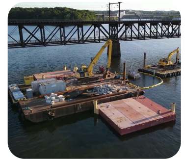
Remnant pier removal
